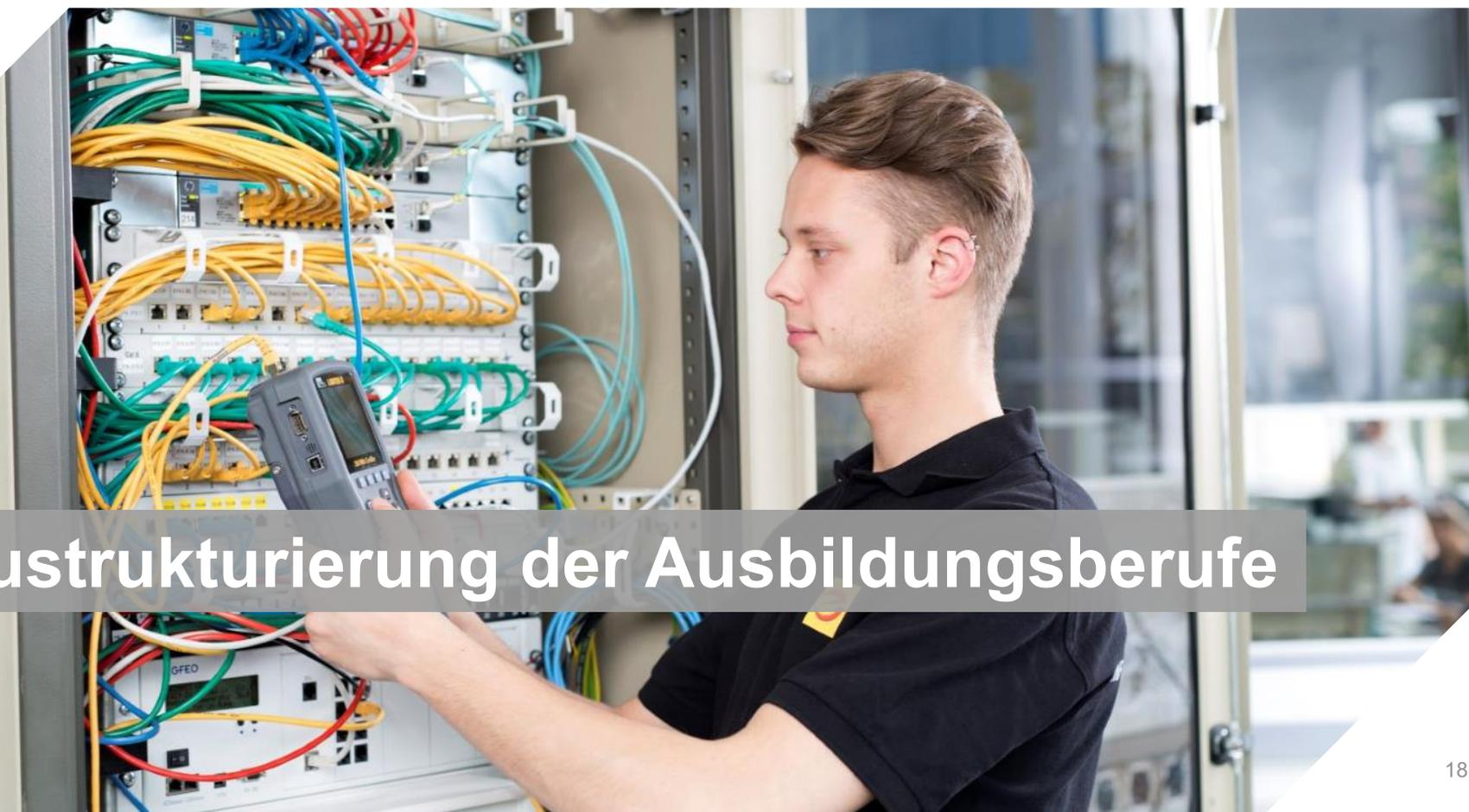
A young man in a black polo shirt is working on a server rack. He is holding a network analyzer or similar diagnostic tool connected to the network cables. The rack is filled with various network equipment and a dense array of colorful cables (yellow, green, blue, red). The background shows a blurred office environment with other people working.
