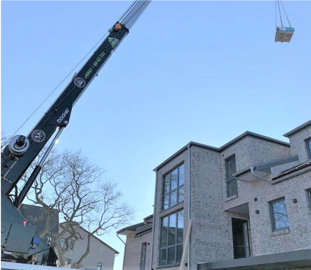
MFH Neubau in Büsum. © Heiwe
